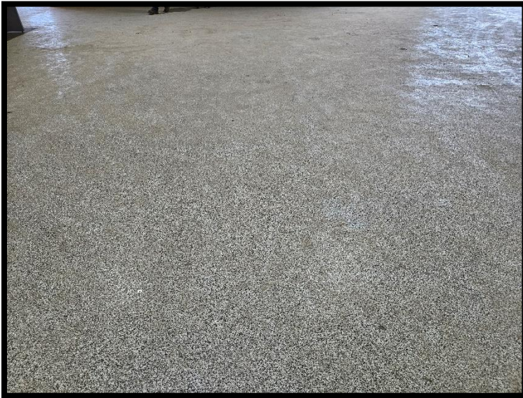
9-Epoxy coating on North half of concrete floor in main building
