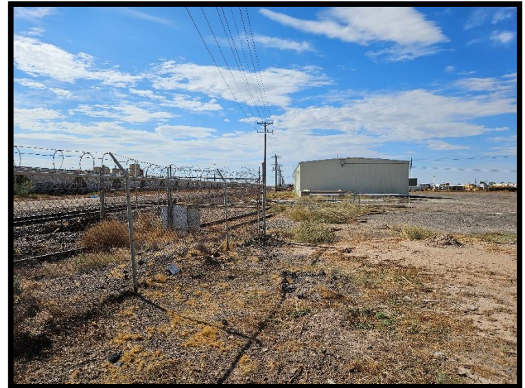
2-View to South from NEC showing former maintenance building (AOC #2)
