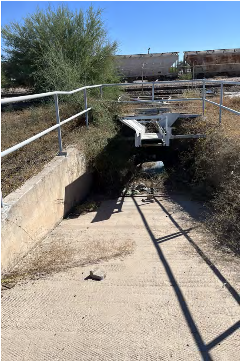
Photo 15: Railcar hopper with unloading conveyor.
