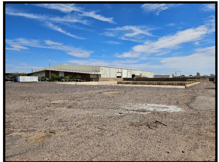
32-View NE of loading dock along S side of building (AOC-5).
