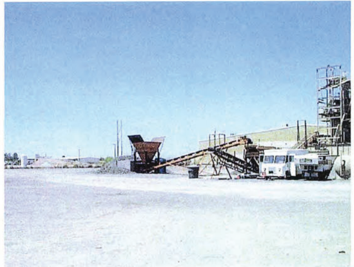
Photograph 6 - View of the hopper and conveyor off the northeast end of the main building.
