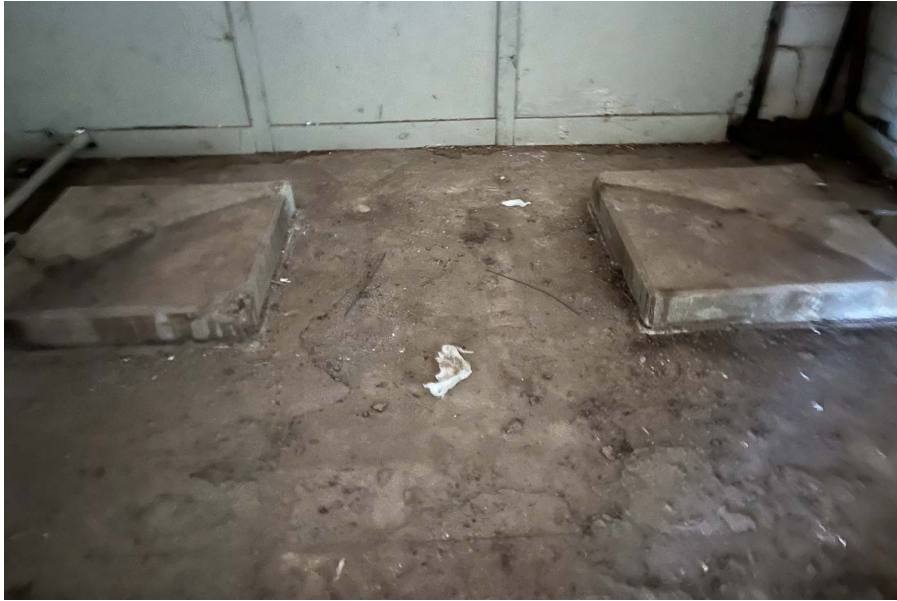
Photo 23: Empty back room in small manufacturing building.
