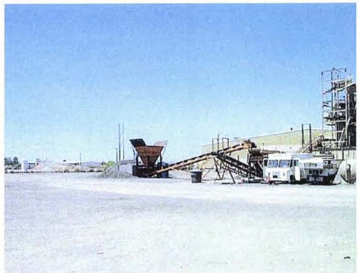
Photograph 6 - View of the hopper and conveyor off the northeast end of the main building.
