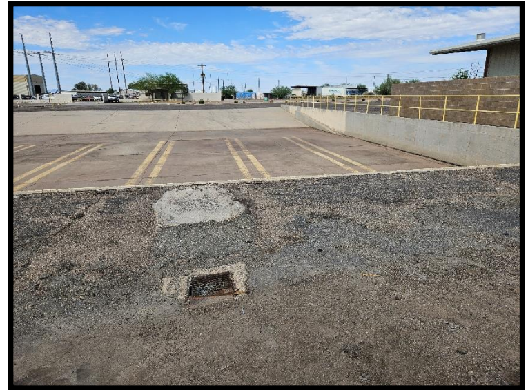
14-Grated drain top of loading dock looking west
