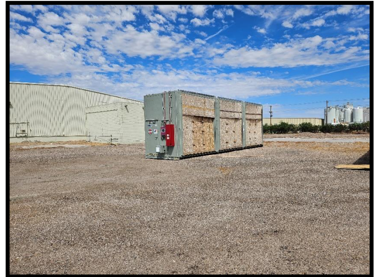
20- View to NW of one normal-risk containment building (SWMU #4)
