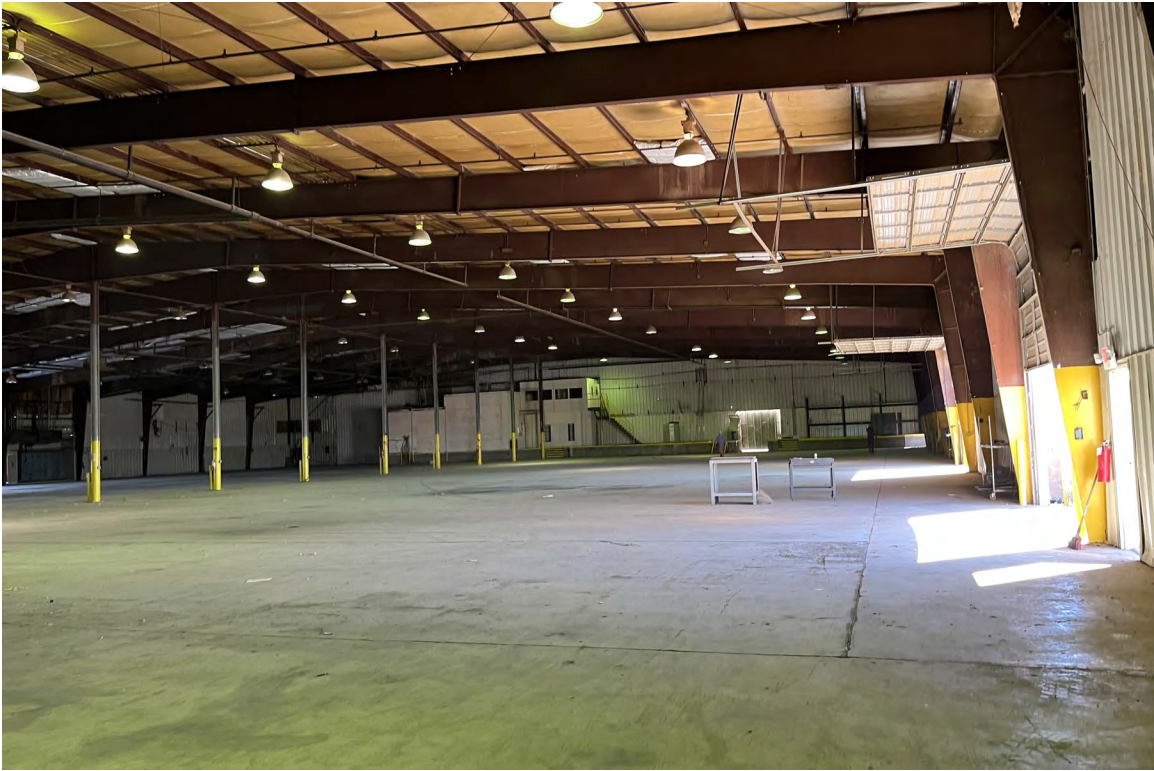
Photo 9: Inside the main manufacturing building.
