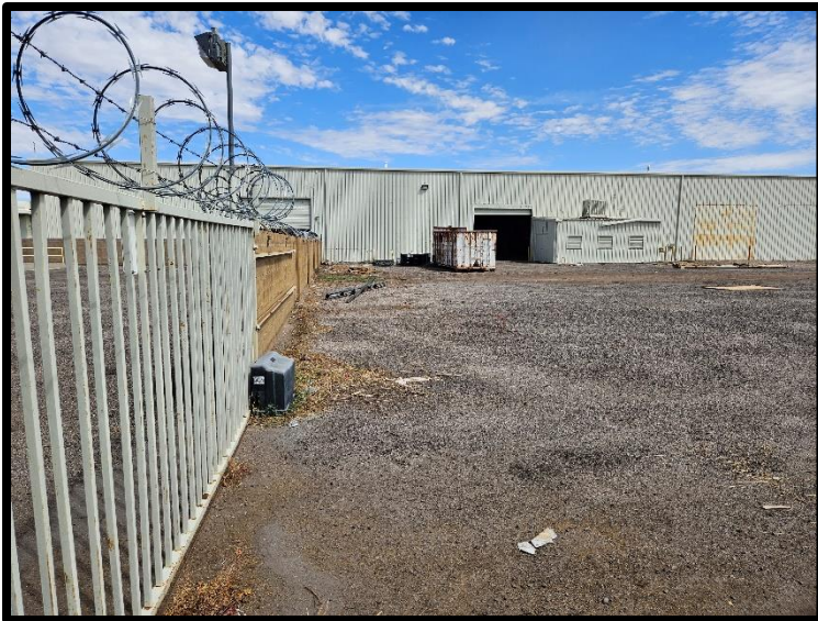
15-East side of security gate along S side looking North
