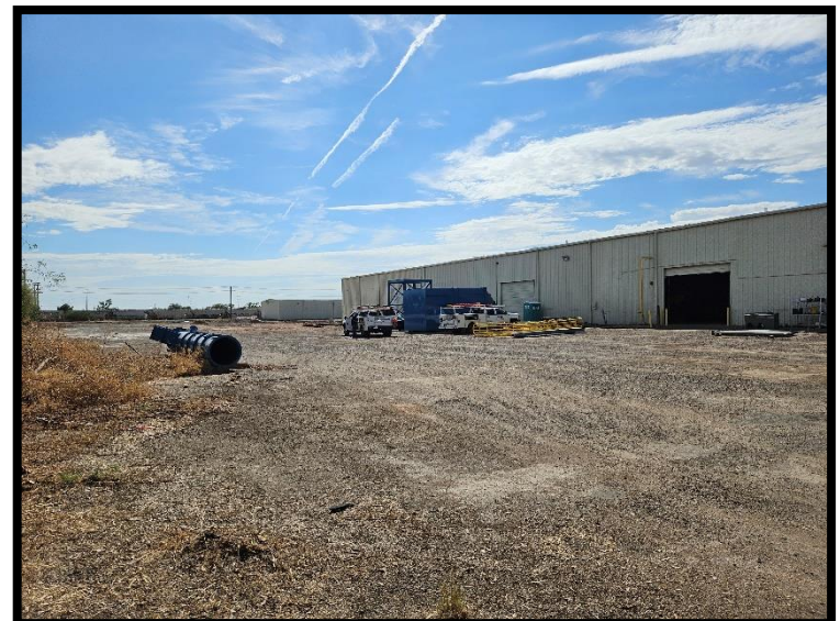
4-View ESE of N side of main processing building
