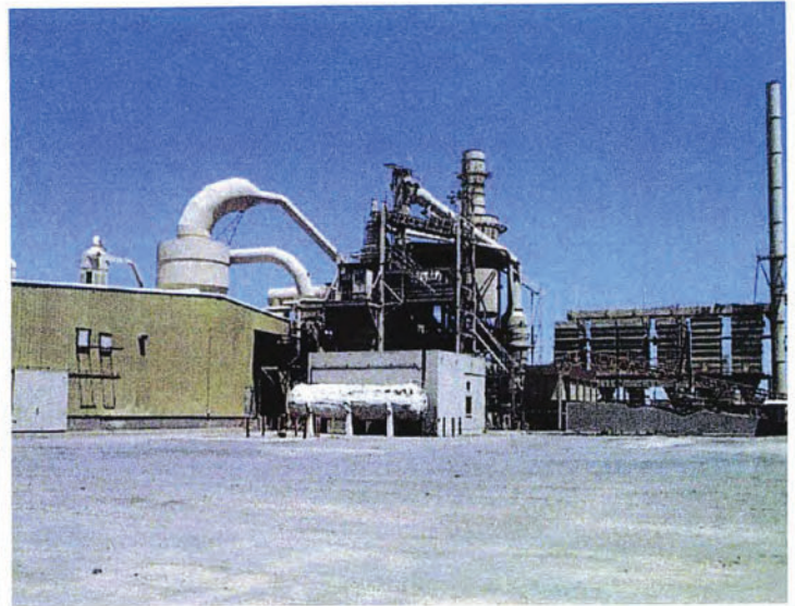
Photograph 4 - View of the east end of the main building, looking northwest.
