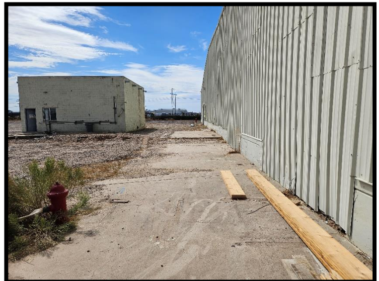
24-View south from NEC of warehouse with former AOC #1 (bldg.) to left
