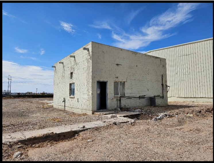
21-View to SSW of reported former fiberglass fabrication building near AOC-1.
