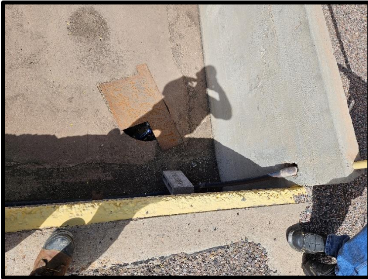
13-View of west drywell (AOC #5) at northwest corner of loading ramp
