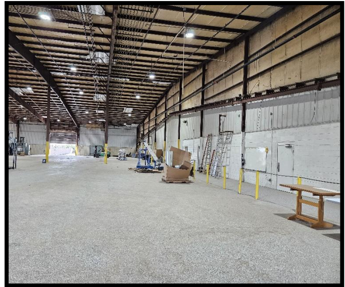
6-View South along W side of main building towards future SWMU #3
