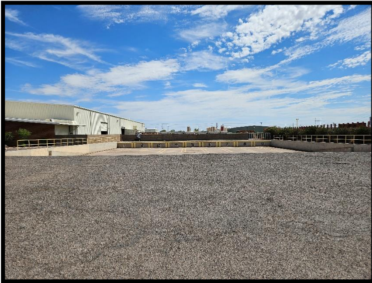
33-View E of 9-lane loading ramp (AOC #5) and dock
