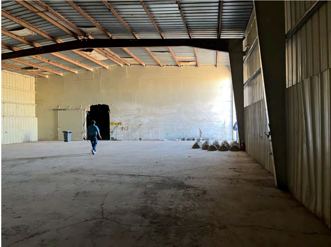
Photo 20: Inside the Warehouse Building.
