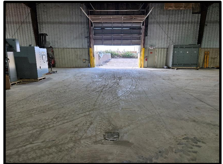
12-Close up of floor drain near west door along south side
