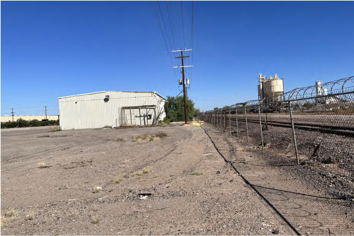
Photo 13: Photo from the southeast corner of the property facing North. Approximate location of former UST.
