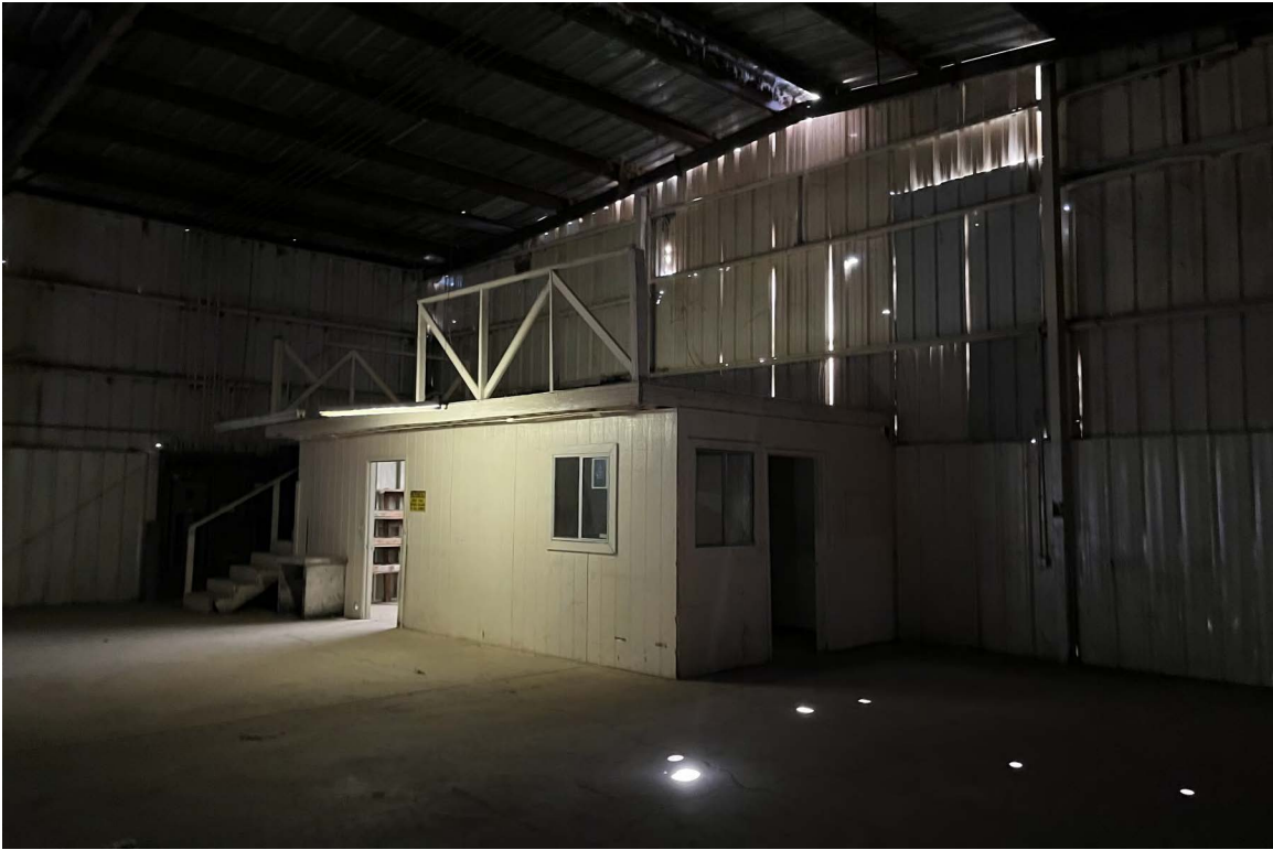
Photo 19: Inside the Warehouse Building.
